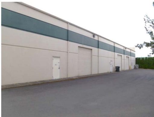
BACK OF BUILDING
